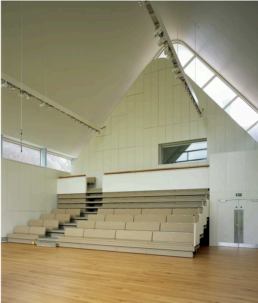
The Recital Hall is designed to provide variable acoustics, with adjustable absorption on the side and rear walls.
