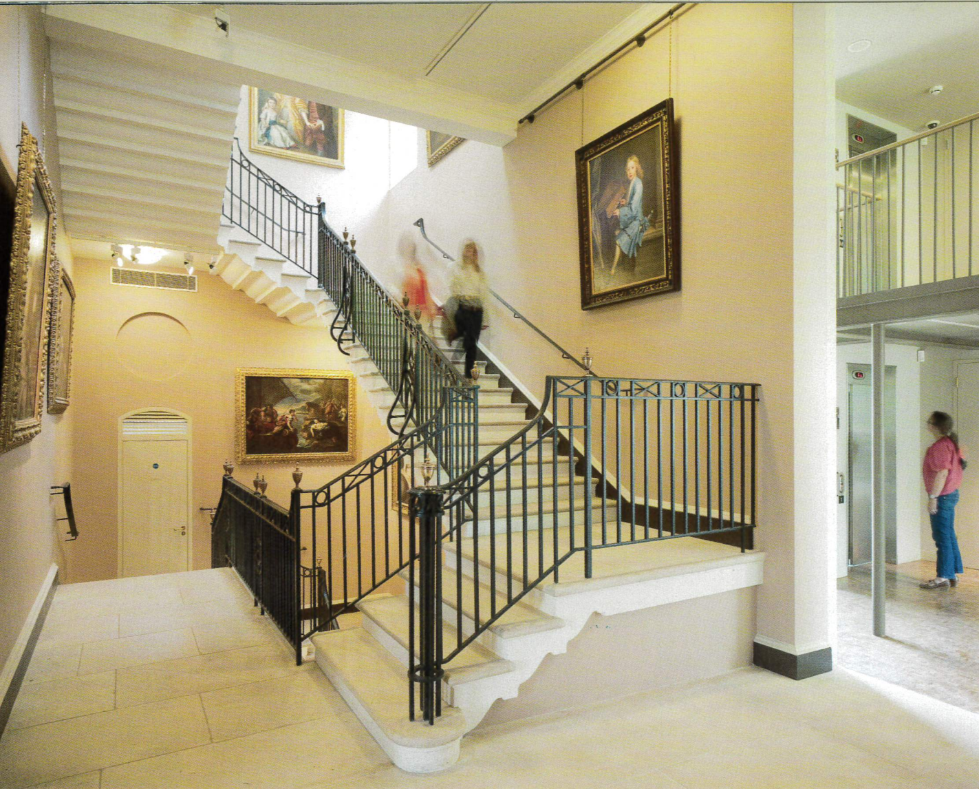
Above The existing main staircase, added when the original hotel was adapted for museum use, was dismantled and moved off centre to allow a central axial route through to the new wing. Left The interstitial link between the old and new buildings incorporates a staircase giving access to the mezzanine level.
