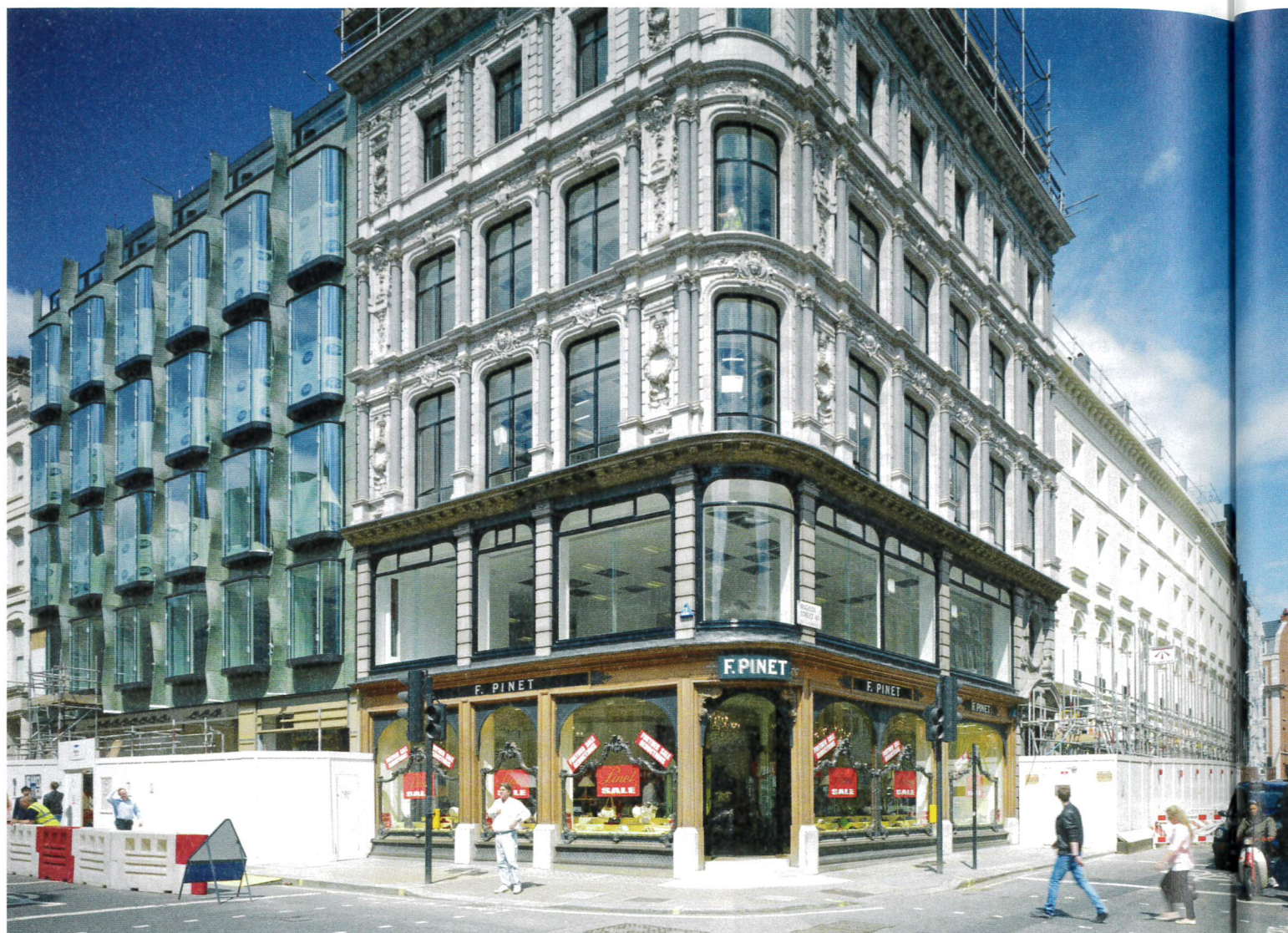
Above The fifth of Eric Parry Architects' London office buildings under construction on New Bond Street. The mixed-use development makes use of both new and existing buildings within an urban block bounded by New Bond Street, Maddox Street and St George Street. A different facade order has been developed for each, including glass blocks and ceramic cladding.
