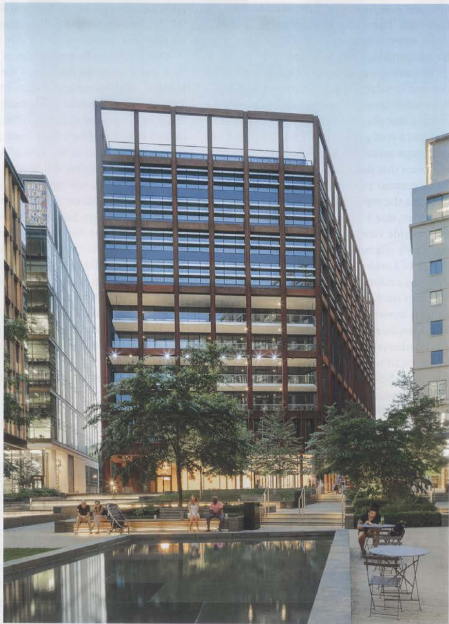
ABOVE 4 Pancras Square mixes weathered steel and ceramic brise soleil
